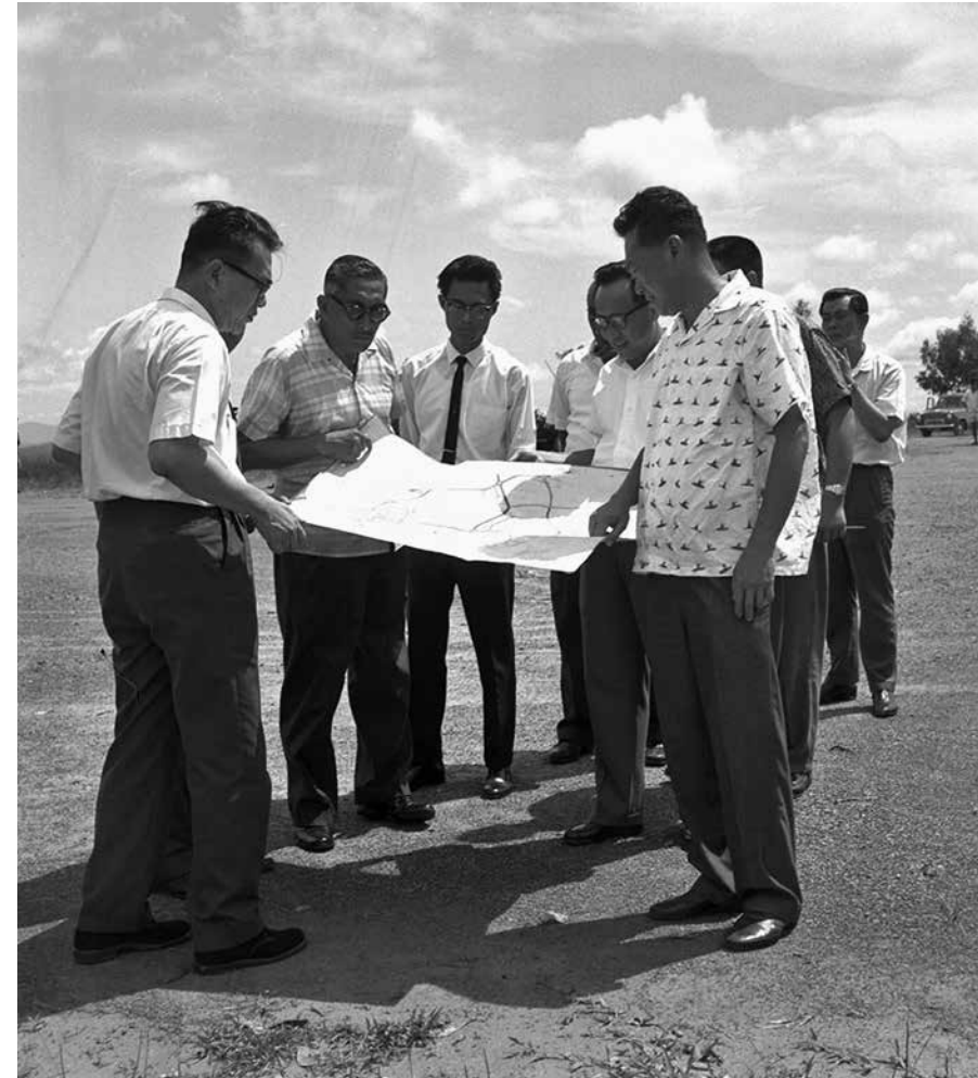
LEFT and BELOW RIGHT: In 1964, Singapore's then Prime Minister Lee Kuan Yew (extreme right); Yang di-Pertuan Negara Tun Yusof bin Ishak (second from left); and the Economic Development Board chairman, Hon Sui Sen (extreme left), toured Jurong Industrial Estate. Accompanying Mr Lee on the tour were Mrs Lee and their three children (below right).
